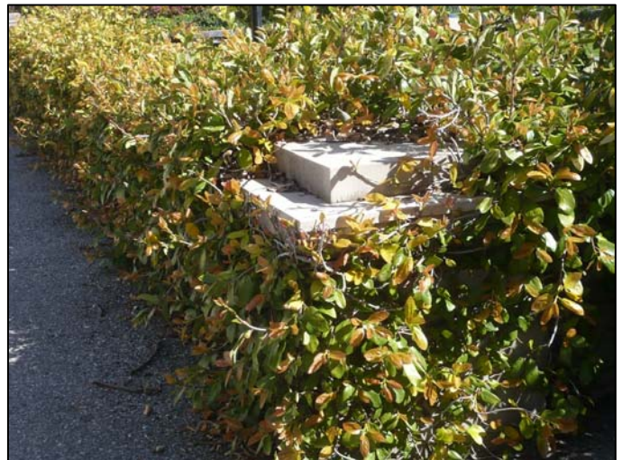
MIDDLE RIGHT: Pedestal of balustrade is barely visible due to overgrown plant material. Such growth must be removed with utmost care, under the direction and guidance of a materials conservator, to avoid damaging the historic material of the balustrade.
