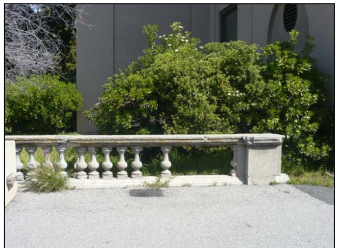
LOWER RIGHT: Short section of balustrade in obvious need of repair and replacement.
