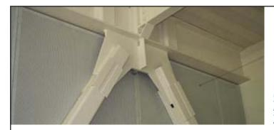
For tension, the exposed braces are reinforced by four angles mounted over the corners of the square HSS brace. These angles provide additional area to prevent a weak section where the brace is slotted to fit over the gusset plate.
